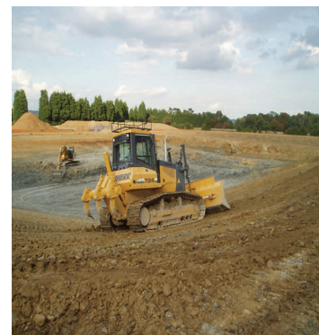
Work underway on the reservoir at Style Place Farm
