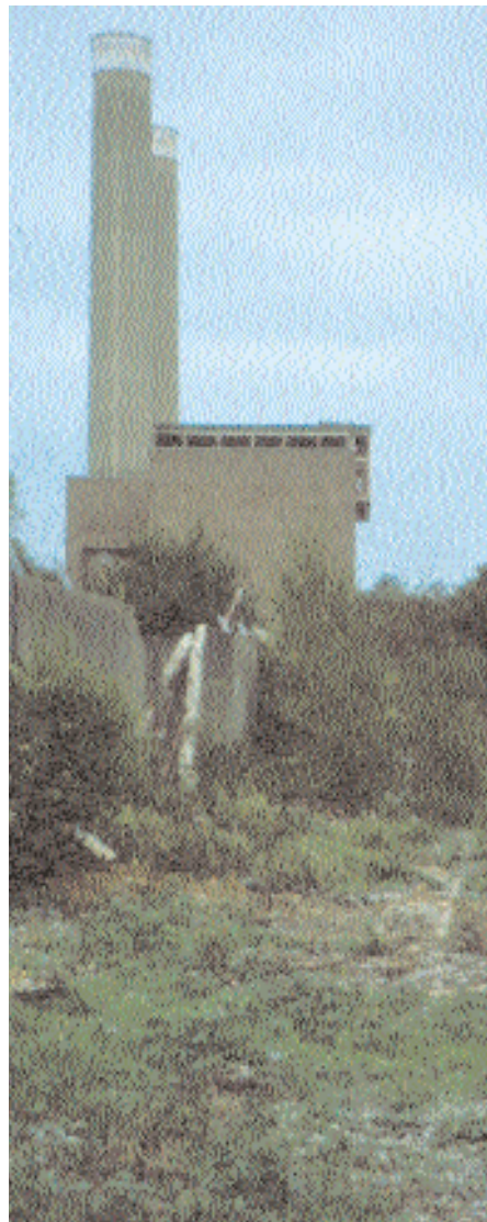
Remaining section of the power station providing a home for common lizards.
