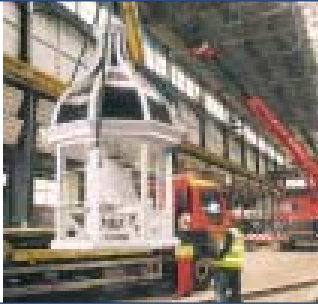
Bell Mast, Chatham Maritime. There are nine Scheduled Ancient Monuments and Listed Buildings at Chatham Maritime under SEEDA's care. In 2000/1 SEEDA renovated the 120 year old wrought iron Bell Mast, which weighs over 20 tonnes and stands 100ft tall.
