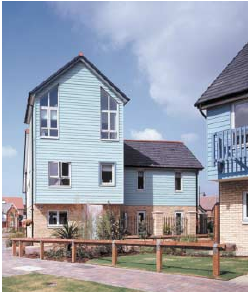
Chatham Maritime - SEEDA's flagship regeneration project - is one of only three schemes in the UK comprising of over 100 houses with 'BREEAM EcoHomes rating'.
