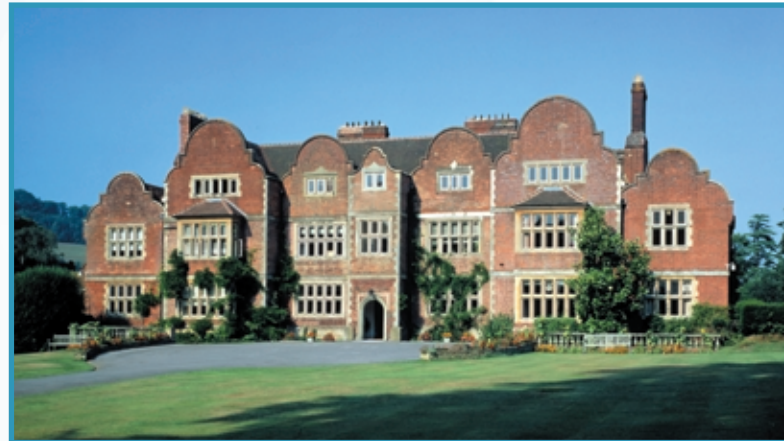
UnumProvident's Head Office, Milton Court, Dorking, Surrey a Grade II listed building
