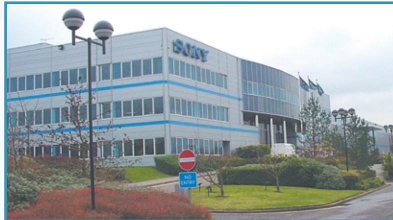
Sony Offices in Weybridge, Surrey. Landscaping is a key feature of all Sony offices, helping to create habitats for, and therefore encourage the presence of, local wildlife
