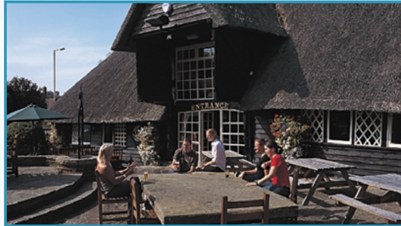
Renovation of thatch at Chestfield Barn, Whitstable, Kent
