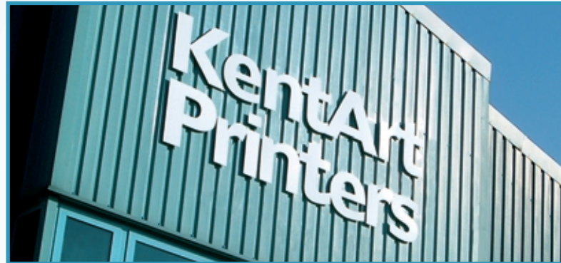
The KAP Factory, Kent
