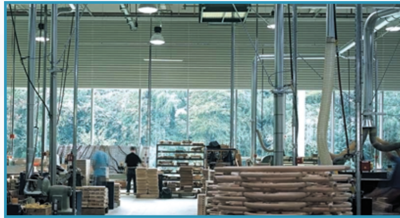
The west facing solar control glass window extends the entire length of the production area
