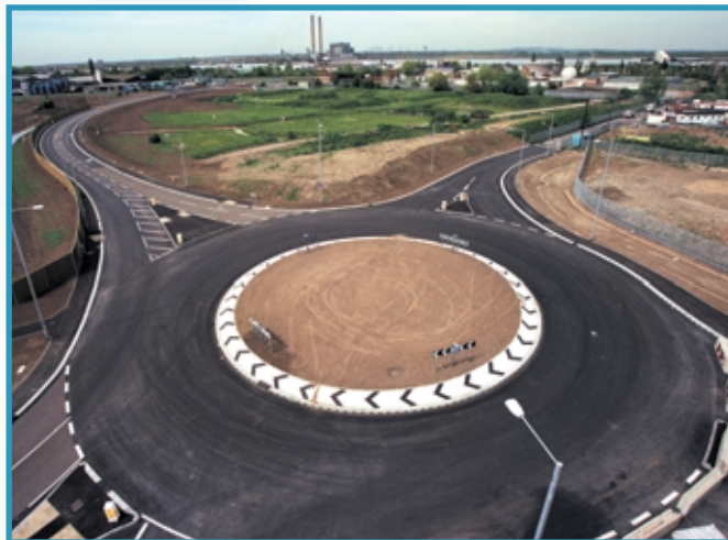
Denton Relief Road, Kent, completed
