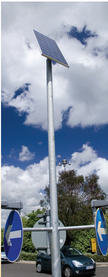
• Solar panel on the airport roundabout
