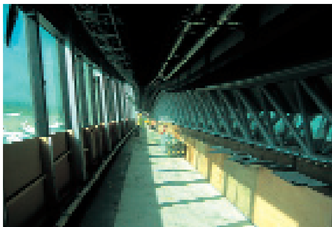
An innovative 'Life cycle' approach was taken on the Pier 6 Project, which has delivered cost, environmental and social benefits
