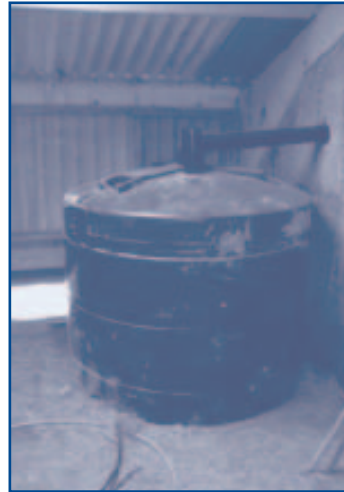
Farm Harvests Rainwater! Jane Howard of Coopers Farm is saving £330 p.a. and 227m 3 water each year. Jane said, "With each cow drinking up to 20 gallons of water a day this soon mounts up in terms of water use and money. So collecting the rainwater pouring down on the barn roofs seemed a brilliant but simple solution to a watery problem... now there are no complaints on this farm every time it rains!"
