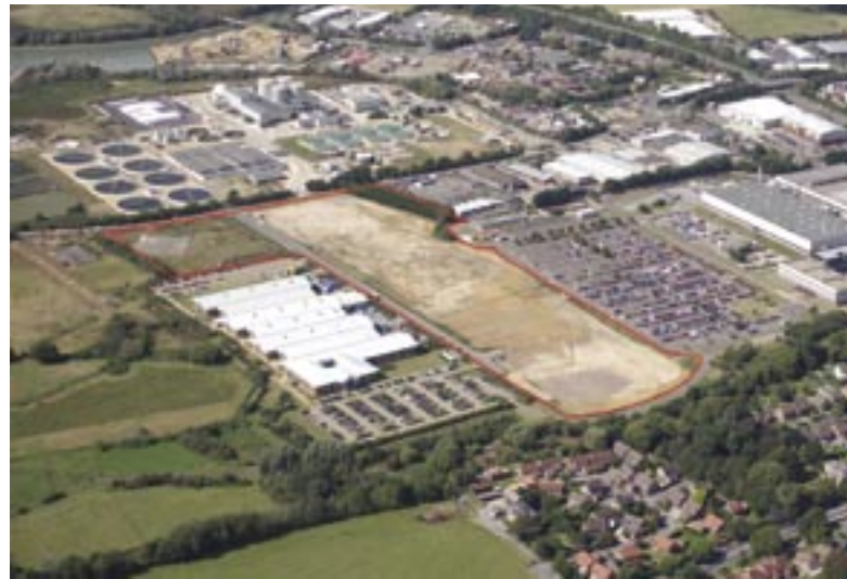
SEEDA has invested circa £4 million in acquisition, reclamation and servicing for Southmoor Park in Havant. The first phase is being developed with Priority Sites for the construction of 7,400 sq. m. of office and industrial units. The remediation of phase two is underway with 2.3 hectares being prepared for sale to developers or owner-occupiers. The final phase will be sold to Havant Borough Council as a site for their new transport and waste-recycling depot.
