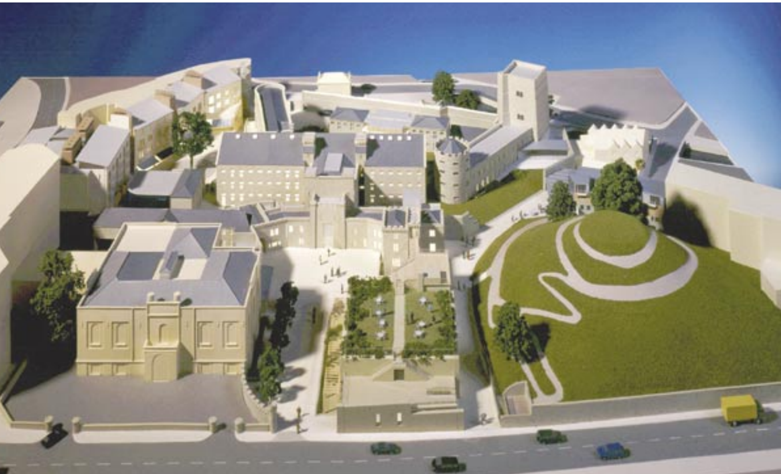
The Oxford Castle and Prison Projects are flagship urban renaissance projects for SEEDA. The picture shows a model of how the scheme may look on completion in 2005.
