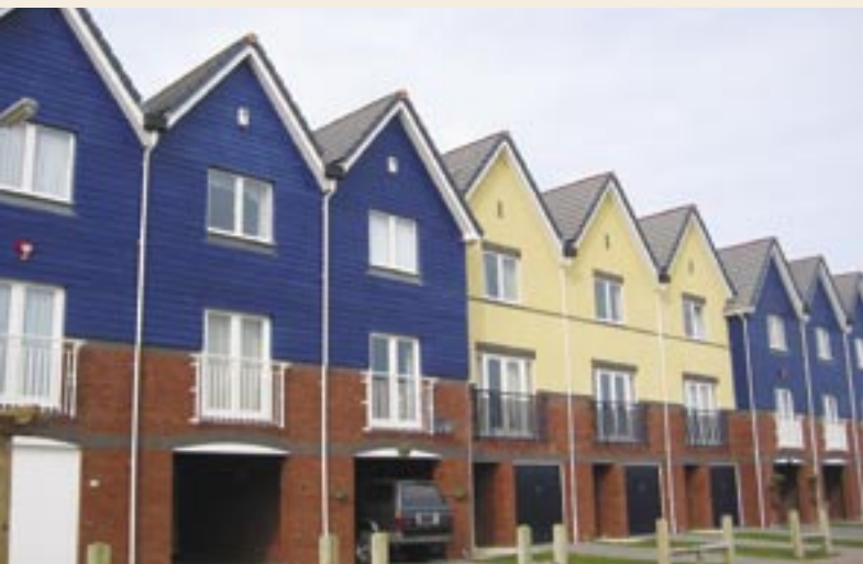
Housing at West Quay, Newhaven, East Sussex - SEEDA's £2 million contribution enabled this high quality mixed-use scheme to go ahead.
