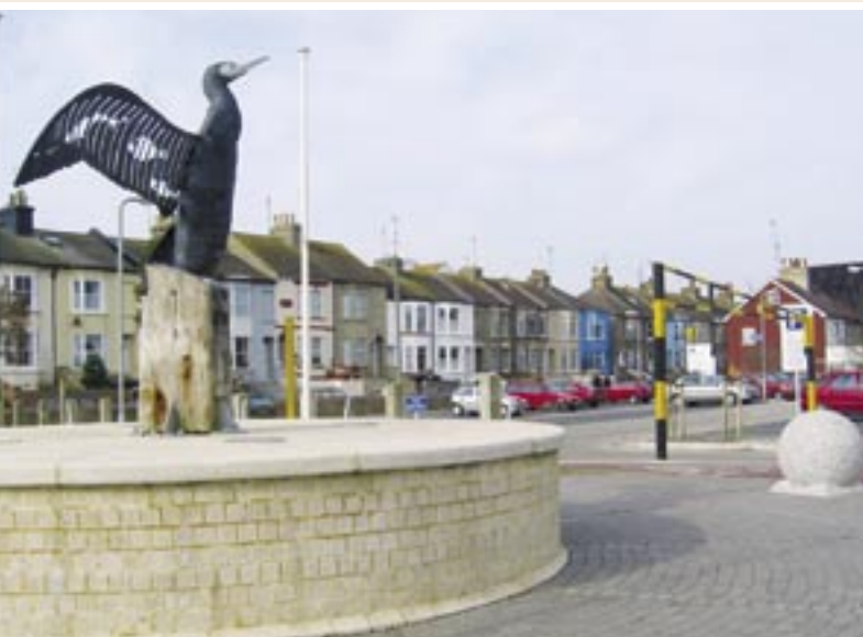
Public realm improvements, part of the SEEDA-funded West Quay development in Newhaven.
