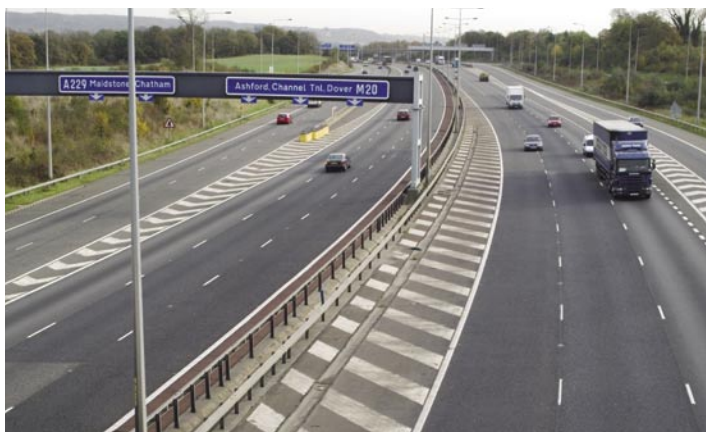
Transport congestion is a challenge for the South East with increased traffic, and longer travel to work times. SEEDA is working with partners to deliver integrated transport and development schemes of strategic national and regional value.
