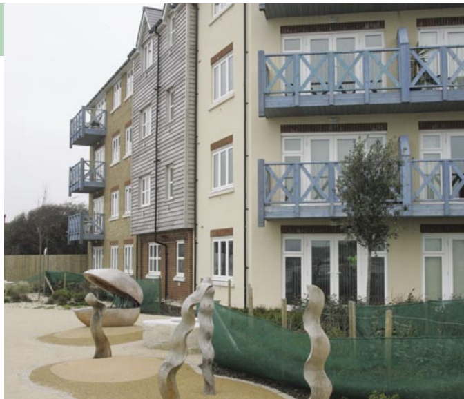
At the centre of the Ropetackle scheme is a new town square, linked to a series of public open spaces with a new riverside walk. This mixed-use development comprises of both residential dwellings and dedicated business space.
