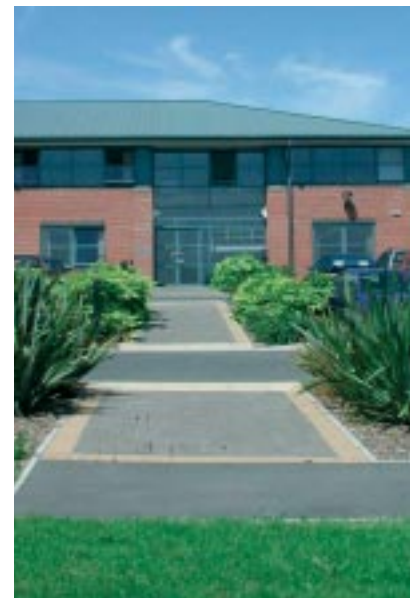
Innovation Centre at St Cross Business Park on the Isle of Wight
