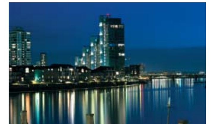
Montevetro, London. Architect: Richard Rogers Partnership.
